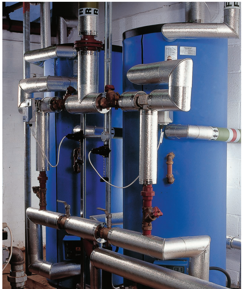
Modular installation of Powerstock calorifiers
